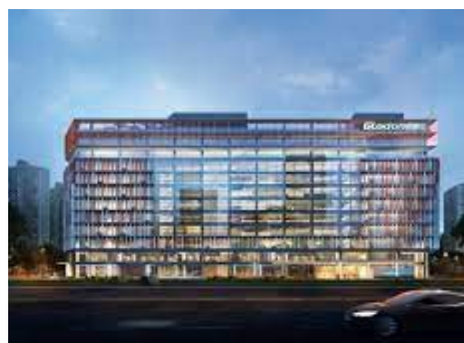
Glodon (Xi'an) Digital Building R&D Mansion Tower
